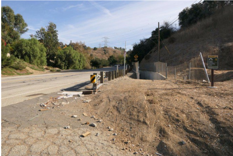
Photo 1. From the west side of Hacienda Boulevard, any would-be user of the pedestrian tunnel must first ignore the at-grade crossing option and choose to walk down a narrow, 90-foot-long, concrete-sided ramp (at right in this photo) that does not appear to lead to the east side of the road. There is no intuitive reason to expect most animals (or humans) to choose the ramp.
